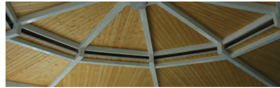
Interior view of Vented roof option
