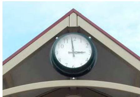
Clock and curved tie beam
