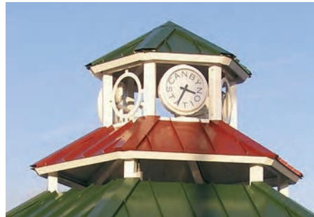
Clock in open steel-framed cupola
