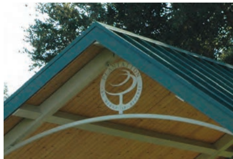
Curved tie beam with laser-cut medallion
