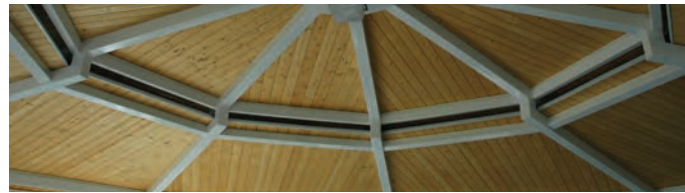
Interior view of vented roof option
