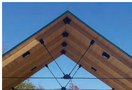
Rod and clevis ties
