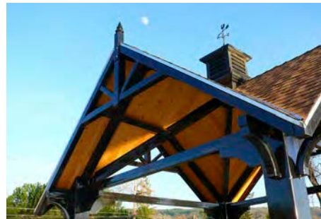
King Post with spire and lower tie beam
